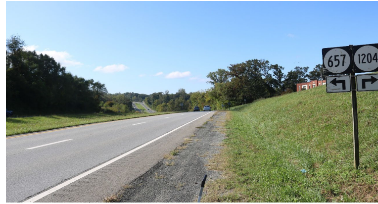
Southbound approaching Rothwood Road
