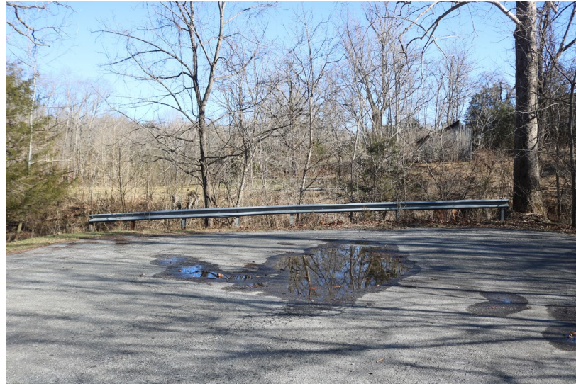
Southbound bridge approach
