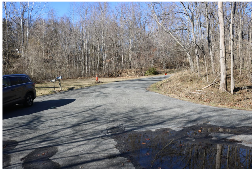
Southbound approach looking north
