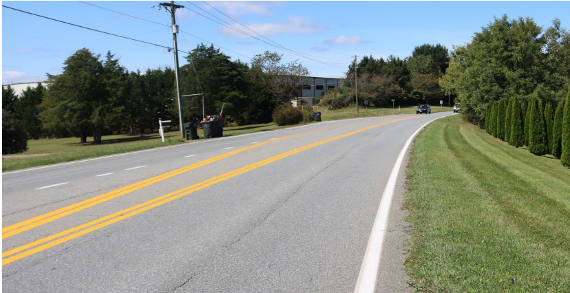
Northbound approaching Mays Mill Road
