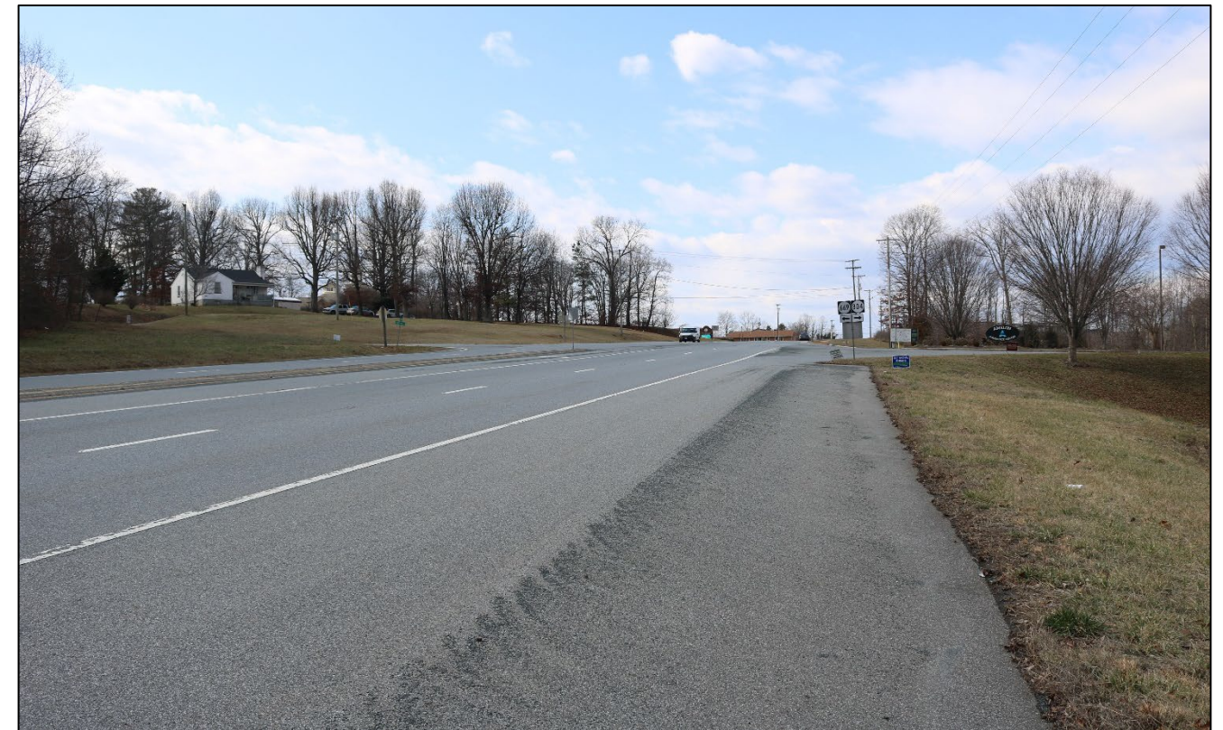
AMELON EXPRESSWAY LOOKING EAST TOWARD AMELON CENTER PARKWAY
