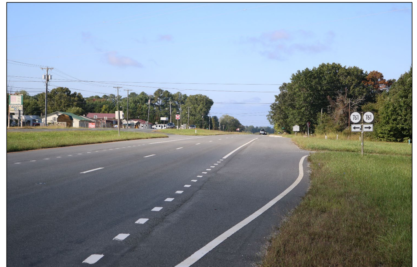
US ROUTE 29 BUSINESS LOOKING SOUTH
