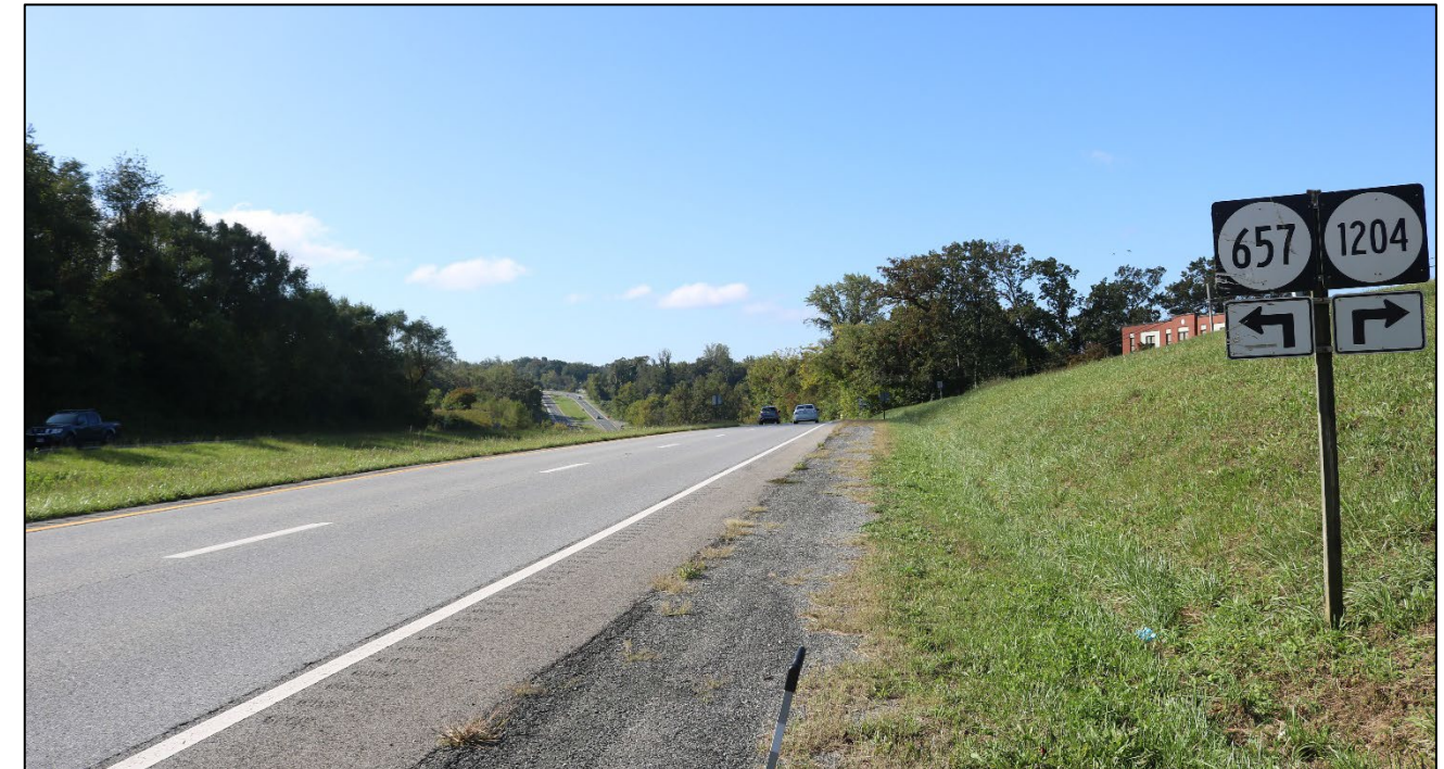
US ROUTE 29 BUSINESS LOOKING SOUTH
