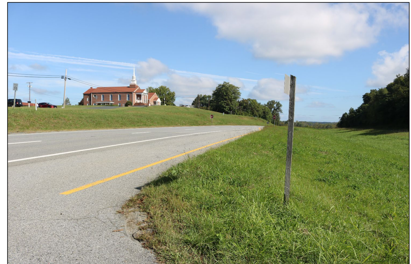
US ROUTE 29 BUSINESS LOOKING NORTH FROM MEDIAN
