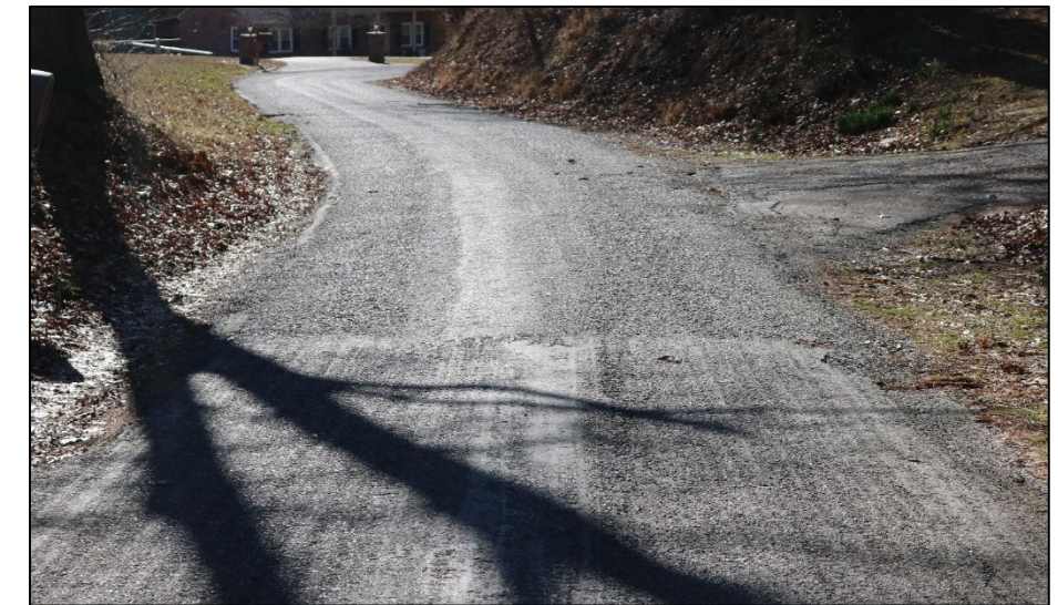
MAYS MILL ROAD NORTH OF FORMER BRIDGE LOOKING SOUTH
